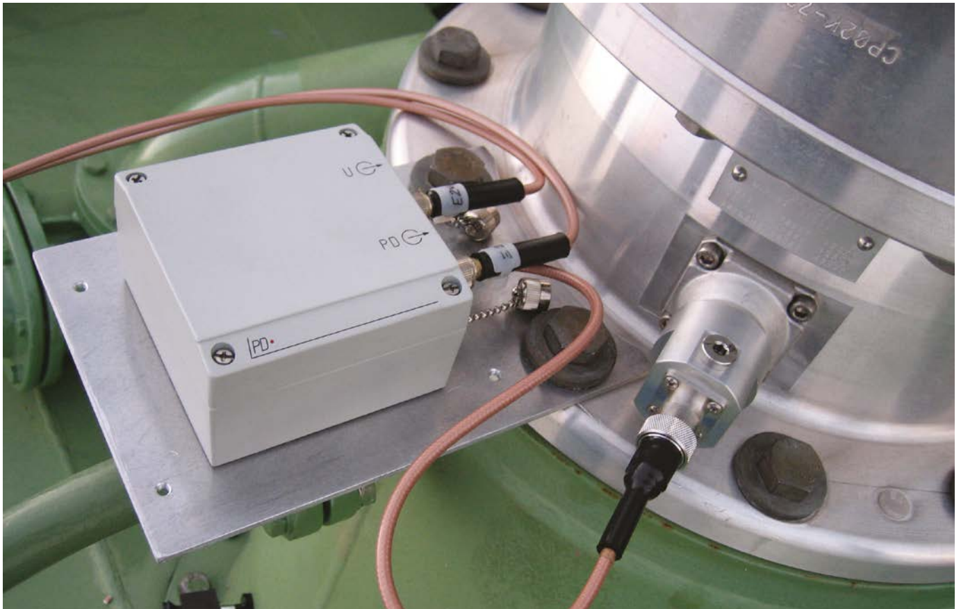
Figure 4. Installed bushing coupling unit and bushing adapter
